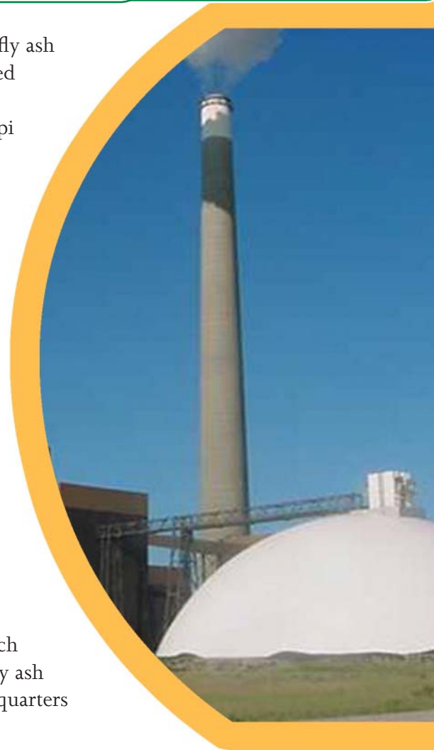
The storage dome collects fly ash from Coal Creek Station in the winter months to meet peak demands during the summer construction season. The beneficial use of fly ash reduces greenhouse gas emissions and the amount of ash disposal at plant site landfills.
